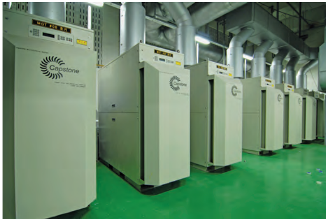
FIGURE 9: Microturbine Installation
